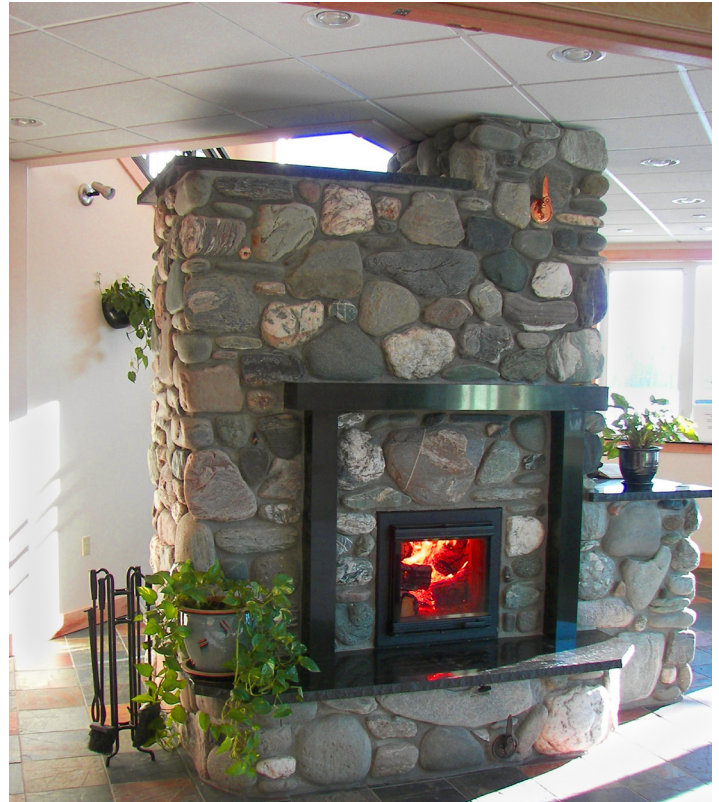
The masonry heater at CCHRC has 12,000 pounds of rock that absorb heat from the fire and radiate it into the room.
