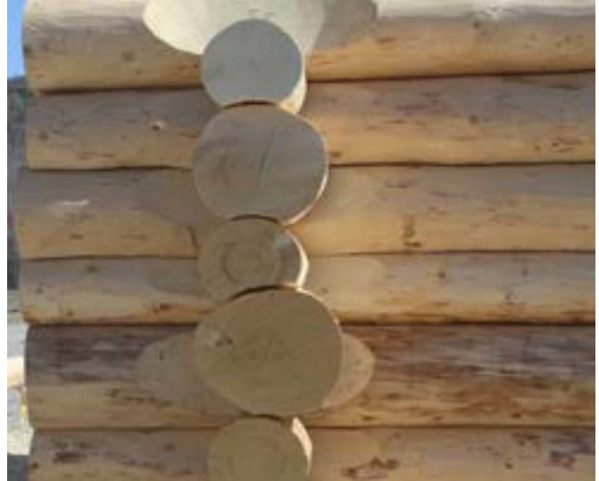
Logs are a construction material with high thermal mass.
