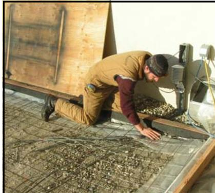
Finishing work on cold weather concrete poured at the west end of the CCHRC Research & Testing Facility.
