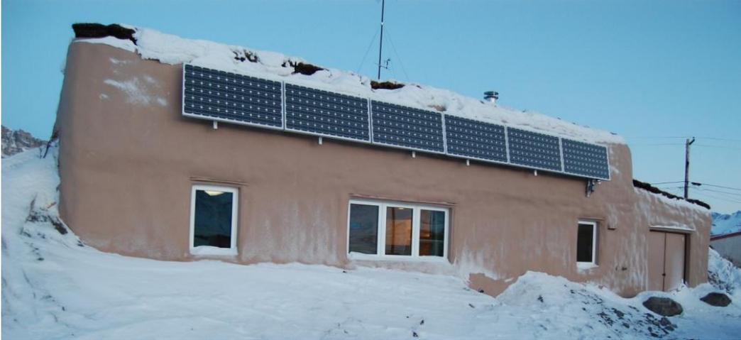
Figure 1. The Anaktuvuk Pass prototype house. The house is earth bermed on the ends to take advantage of the thermal and wind shear benefits of a traditional sod house.
