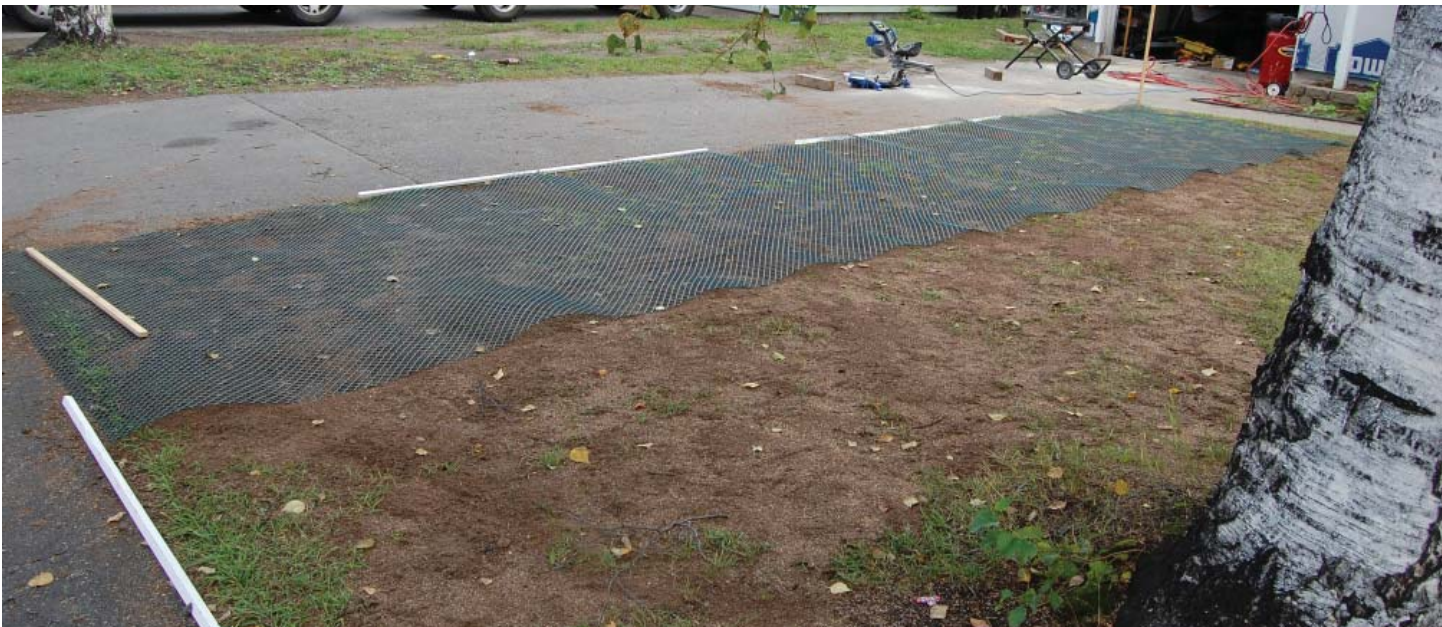
Ground leveled, with mesh laid out prior to pinning.
