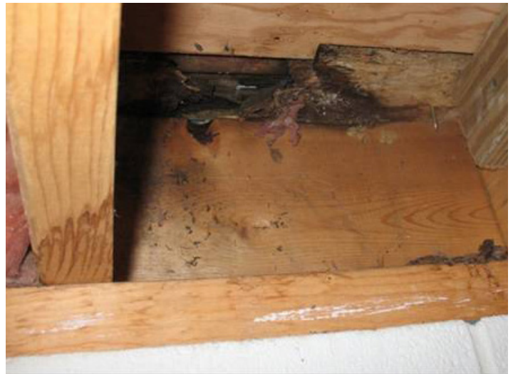
Above: Lack of good sealing and ventilation can lead to mold and rot in the crawlspace.
