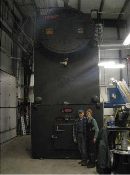
Figure 3: A biomass boiler has been installed to heat the Tok School. Photo courtesy of Alaska Gateway School District.
